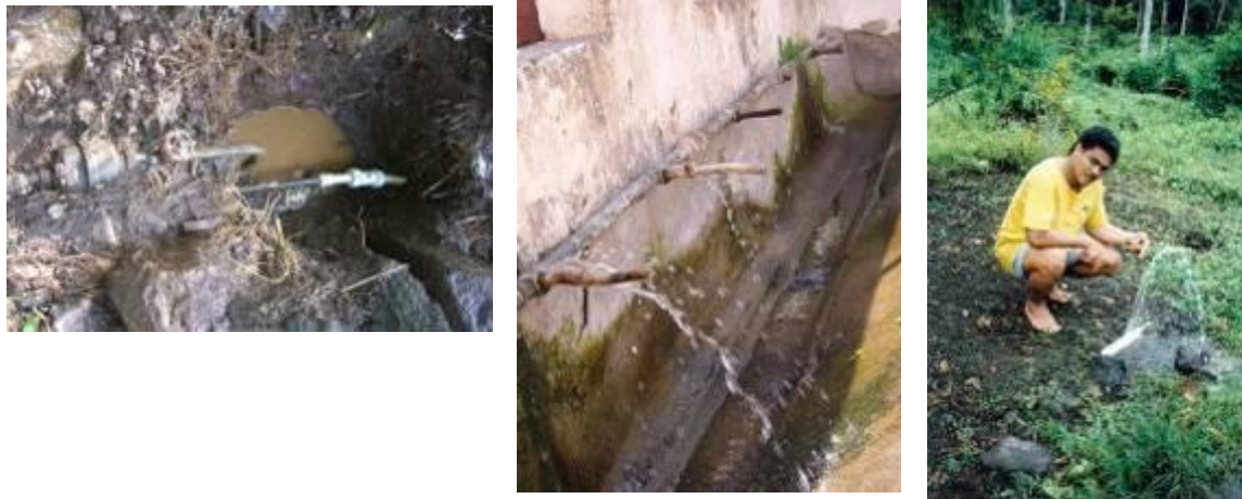
Typically more difficult to detect, service connection leaks result in significant water losses.
