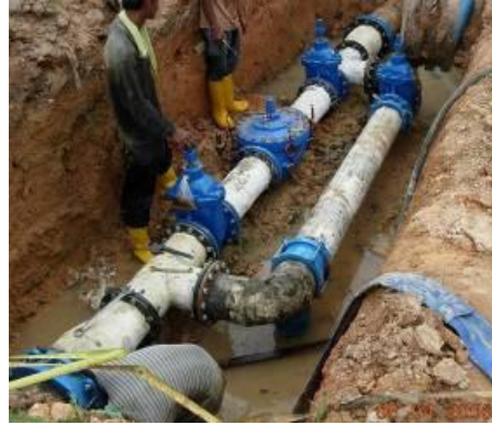
PRVs installed in meter chambers.
