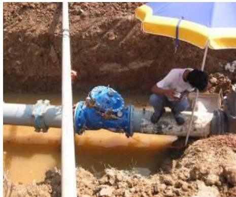
PRVs installed in meter chambers.
