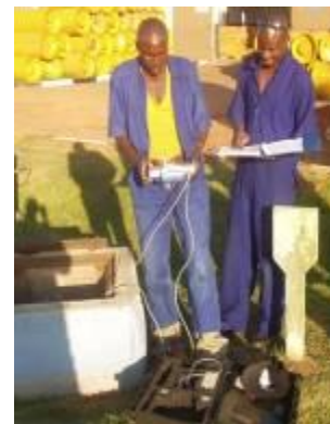
Field verification of the network data is crucial to understanding where water losses originate and setting NRW baseline level.
