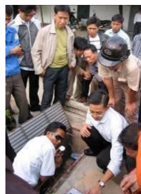
Experts from Ranhill working hand-in-hand with their counterparts in Bac Ninh, Vietnam, to test DMA operations.
