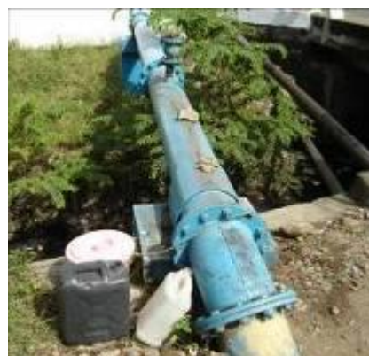
Water theft can occur from large pipes as well as from household water connections.
