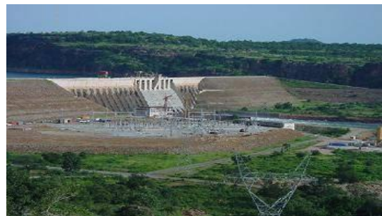
Manantali Regulatory dam (Mali)
