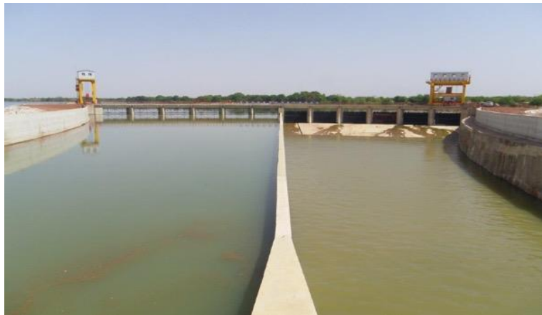
Regulatory Felou dam
