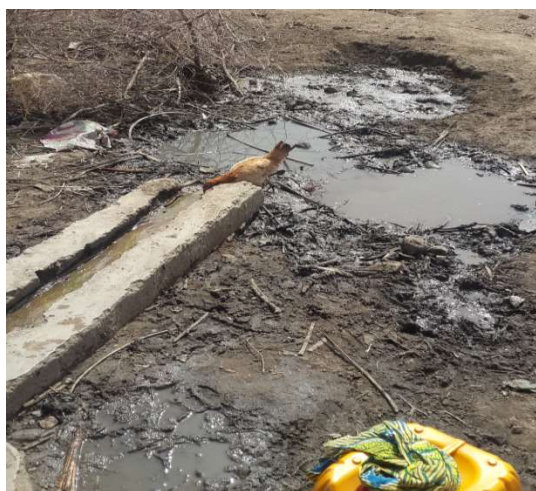
Figure 3.52. Very poor sanitary status at U/Madaki, Dafa Handpump, FCT
