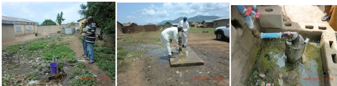
Figure 3.51. Poor Sanitary conditions around some Boreholes in Taraba State.
