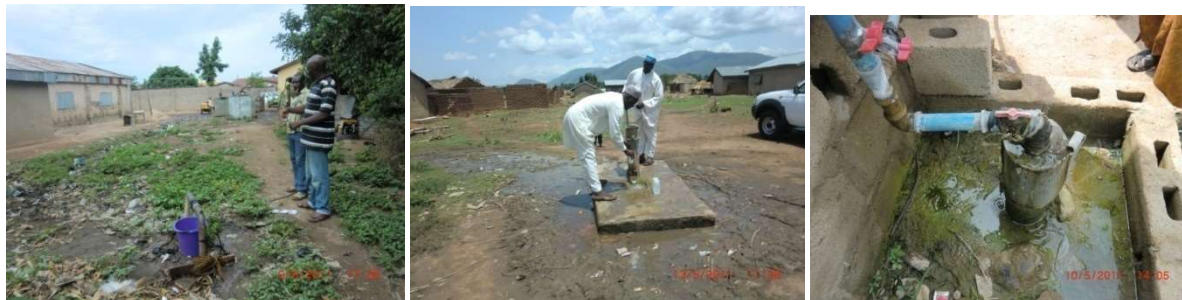
Figure 3.63: Poor Sanitary conditions around some Boreholes in Taraba State
