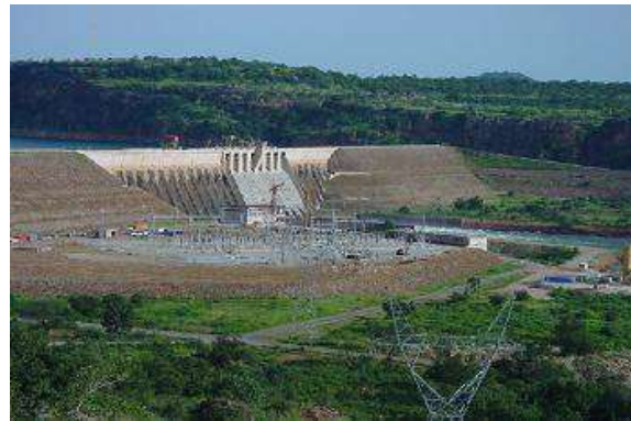
Manantali Regulating dam (Mali)
