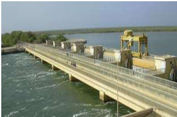
Diama dam Salt barrier (Senegal)
