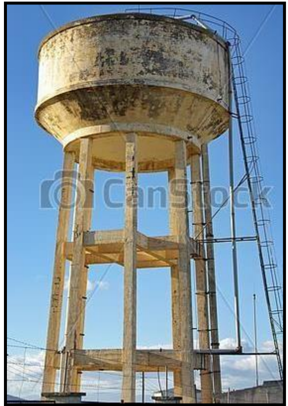
Concrete Elevated Tank
