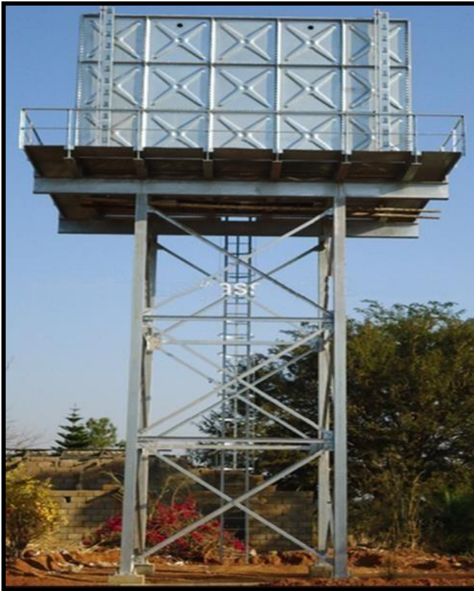
Steel Elevated Tank
