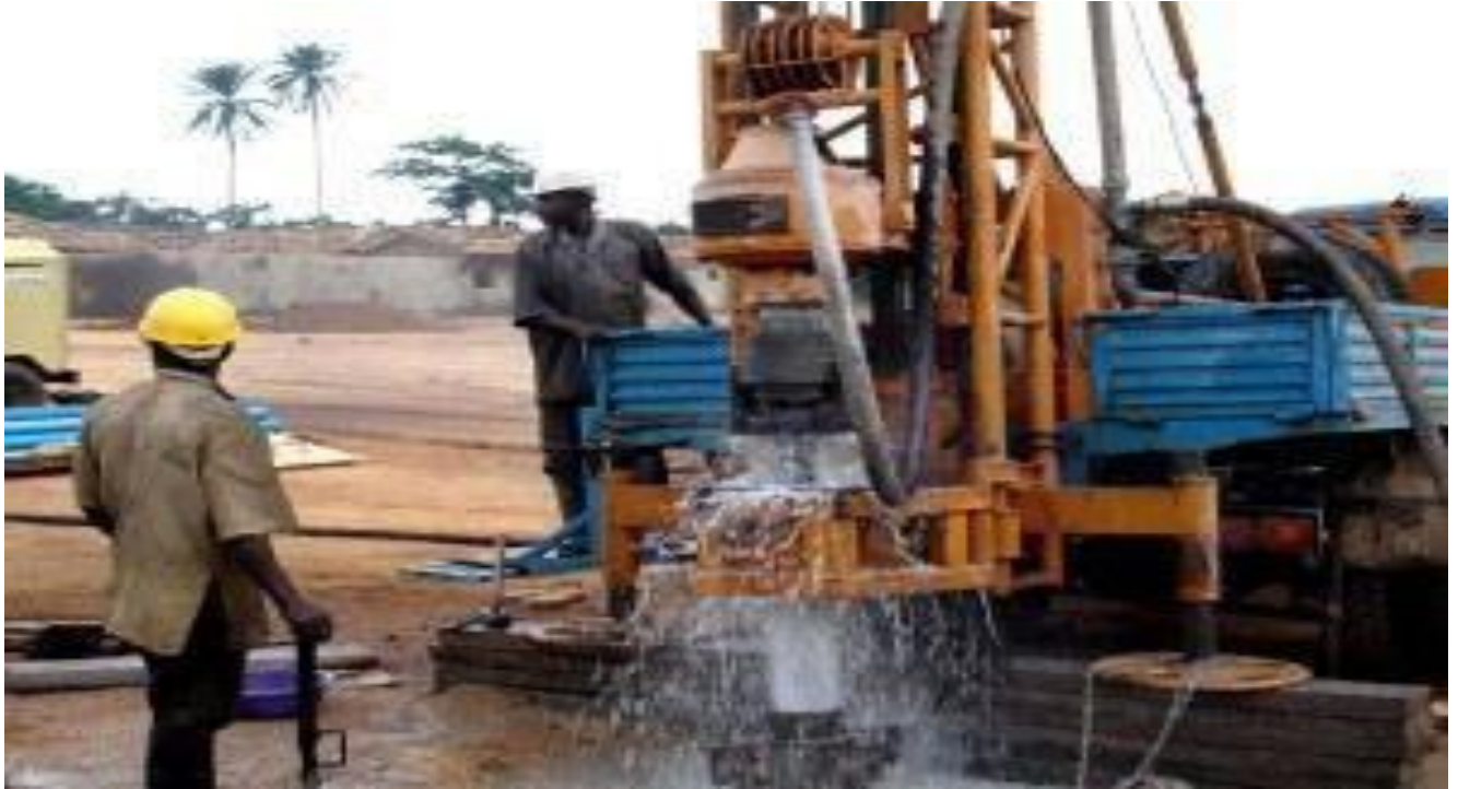
Figure 3: Typical borehole drilling showing water flow
