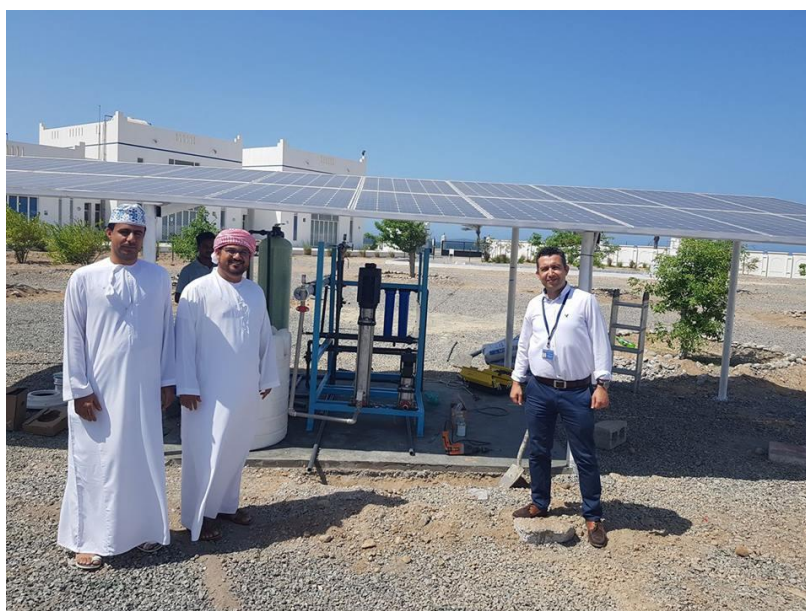
Figure 3. Desalination for agriculture in Oman, project funded by Agriculture and Fisheries Development Fund (RO unit fed by solar PV at MEDRC facilities, North Al-Hail, Oman)
