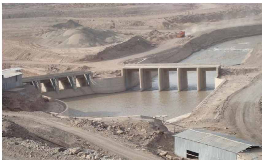
Figure 4. Head regulator of Tandaho irrigation canal and water diversion to the command area.
